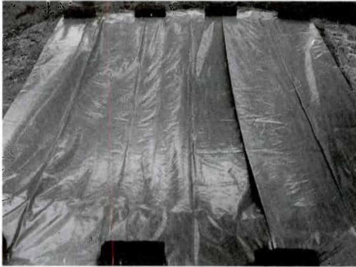
Fig. 2 : Pit covered with a polythene sheet.
